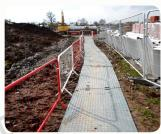
Plastic sheets - surface protection for sports halls, stage floor, ground protection, walkway, mounting floor, edge protection, access road etc. Available in all RAL colors.
